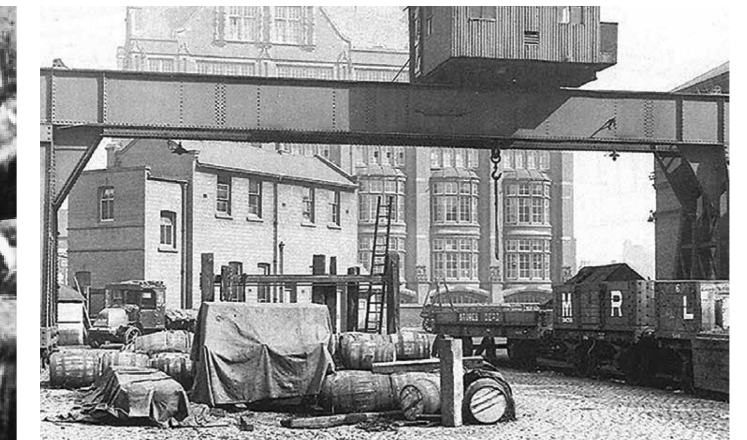
View of the goods yard Goliath overhead travelling steam crane
